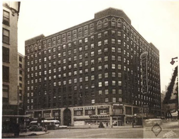
The Empire Building, showing the Riverside Theater (circa 1940's-1950's). B.F. Saltzstein's law offices were on the 14 th floor. https://www.pinterest.com/pin/505106914444427676/
